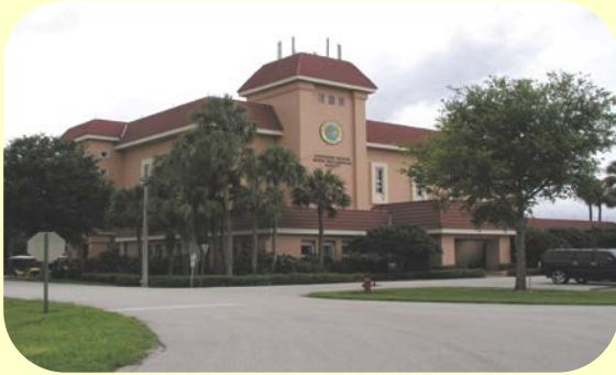
Southern Regional Water Reclamation Facility
