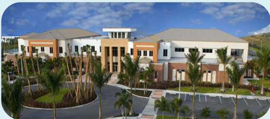
Fire Rescue Headquarters
