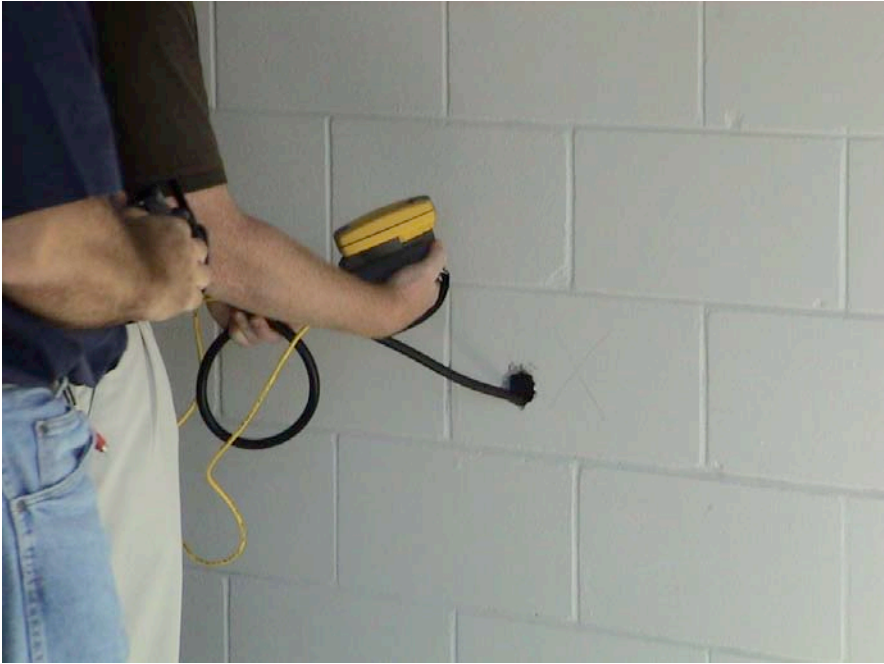
Photograph 45: Camera Probe Leak Detection
