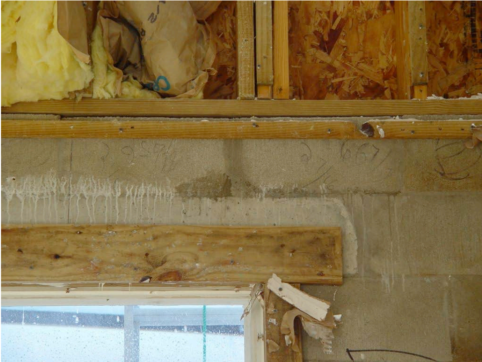
Photograph 17: Water Entry Between Floors
