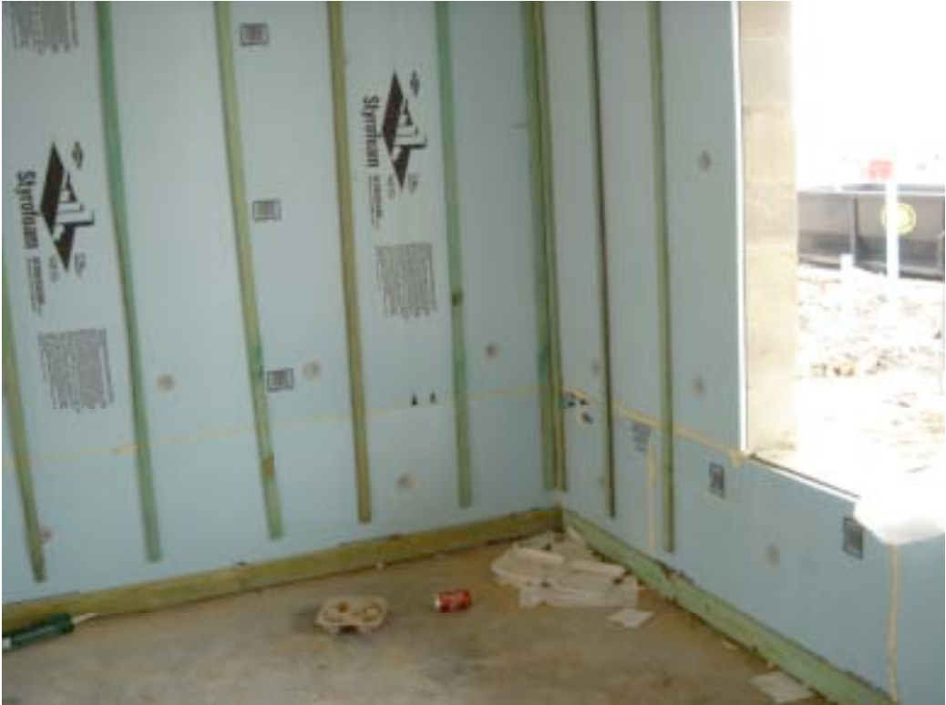
Photograph 64: Rigid Foam Interior Lining Protecting Interior Surfaces
