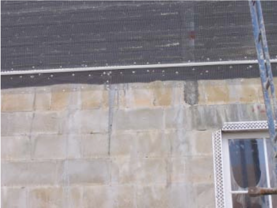
Photograph 17: Water Entry Between Floors
