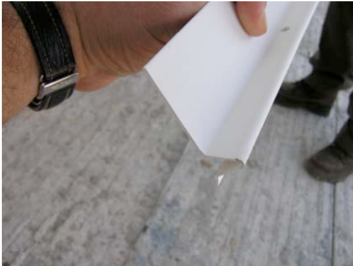
Photograph 18: Flashing/Control Joint - Weep Screed Flashing
