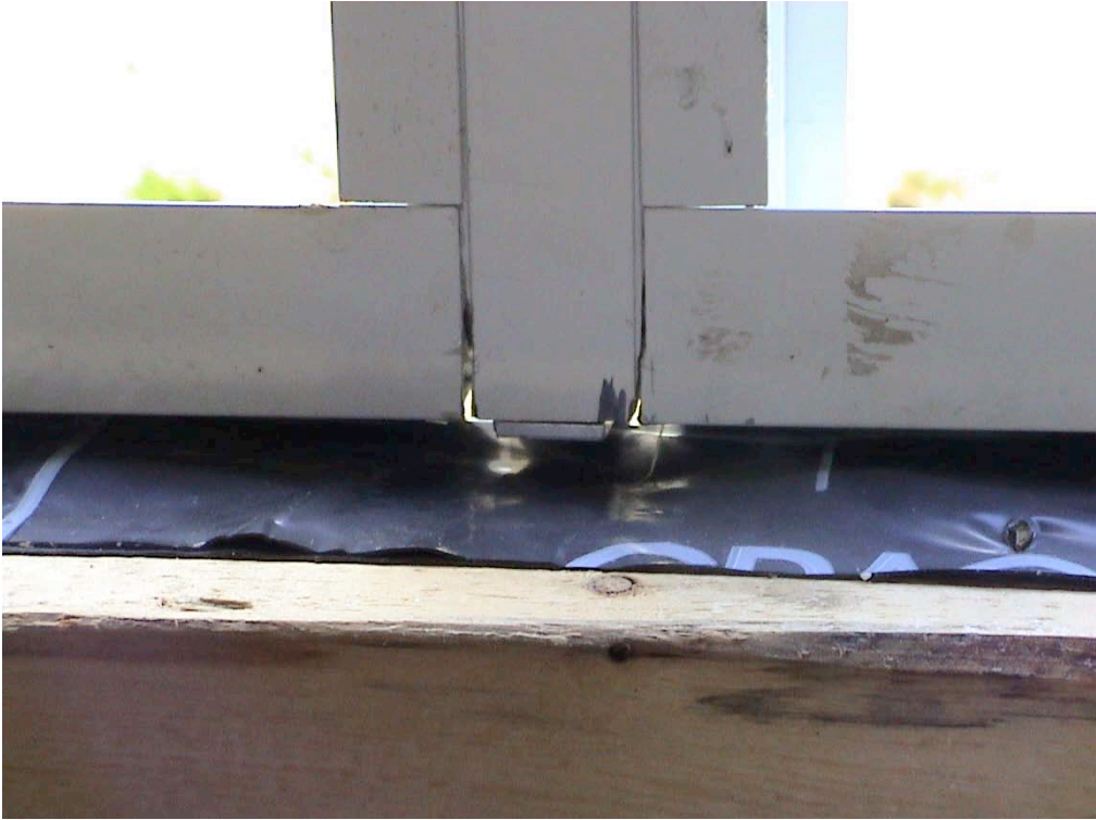
Photograph 26: Mulled Window Unit Leakage Paths
