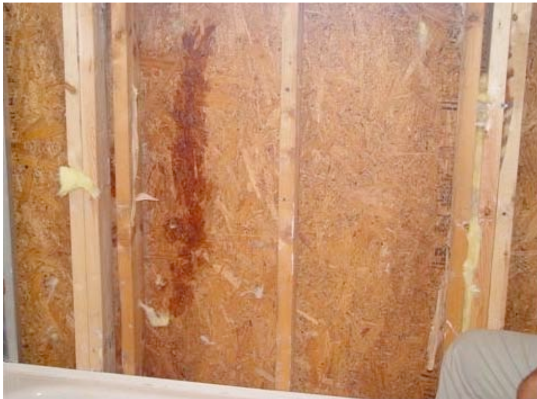
Photograph 2: Rainwater Entry into Second Floor Frame Assembly
