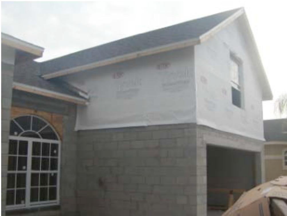
Photograph 13: Enhanced Drainage With A Profiled Plastic Housewrap
