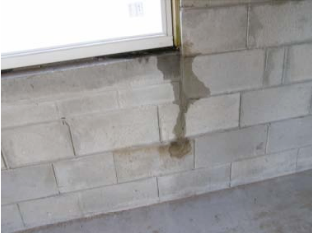
Photograph 24: Window Corner Leakage
