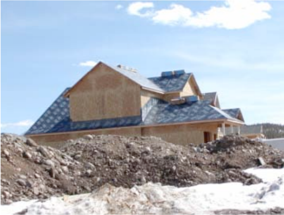
Photograph 72: Direct Applied Self Adhering Membrane
