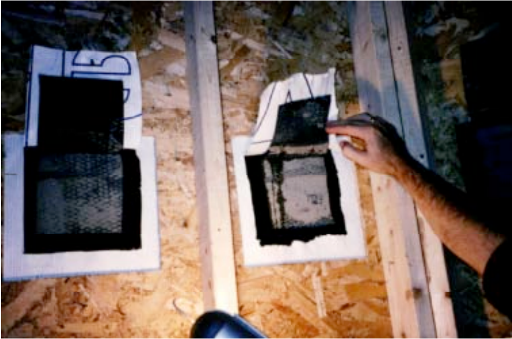
Photograph 12: Paper Backed Lath As A Bond Break
