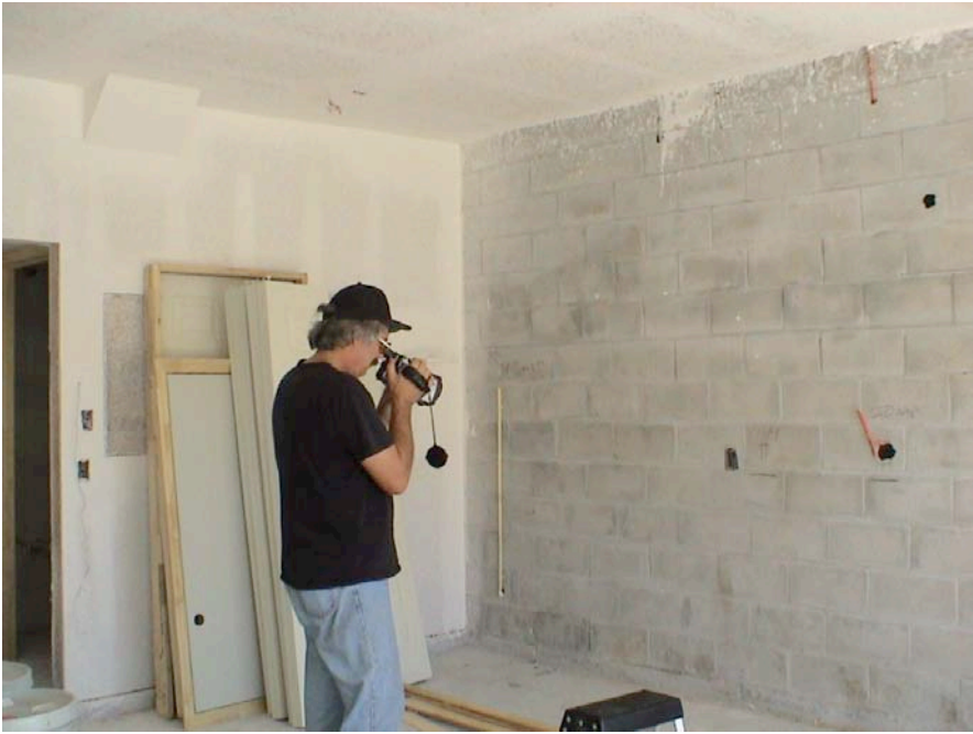
Photograph 44: Infrared Camera Leak Detection
