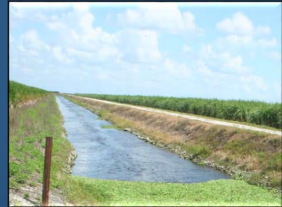
Canal bank vegetation to minimize erosion
