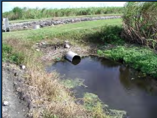
Raised culverts for slower drainage
