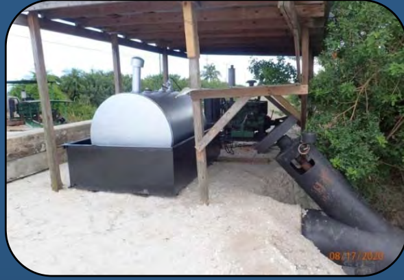
Pump station foundation improvements, fuel tank in protection basin
