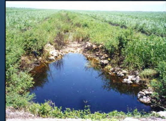
Field ditch sediment sumps/traps
