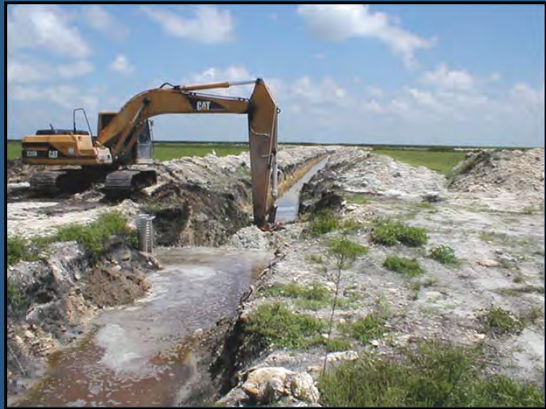
Canal cleaning and capacity improvements
