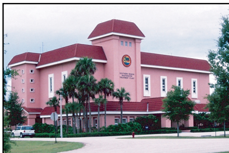
Figure 6-7 Southern Region Water Reclamation Facility
