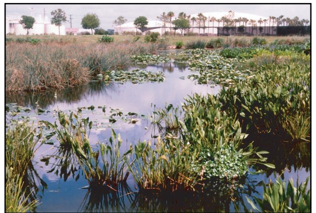
Figure 6-13 Natural Treatment Cells
