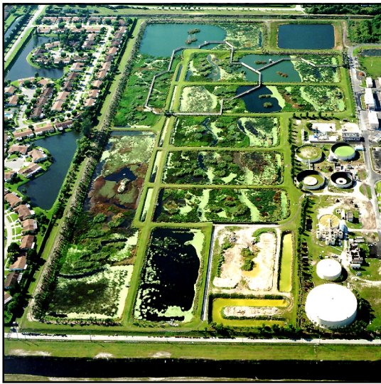
Figure 6-12 Aerial View of Wetlands
