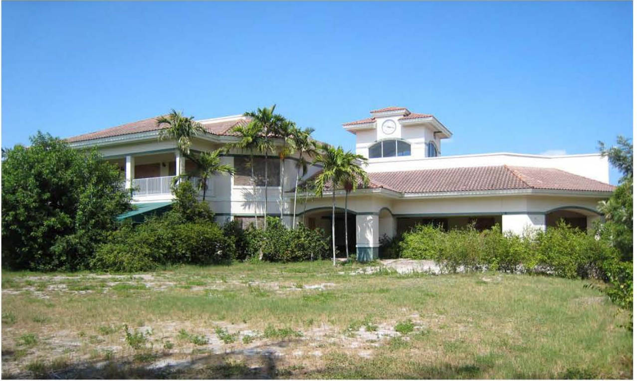
View of Existing Club House
