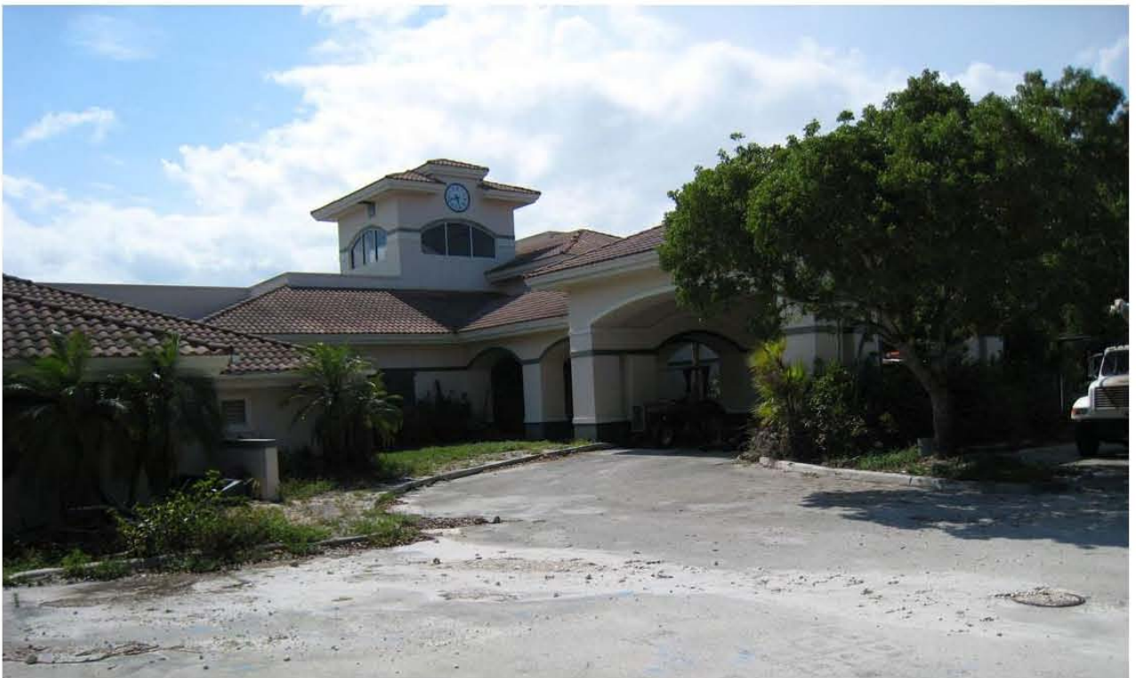
View of Existing Club House
