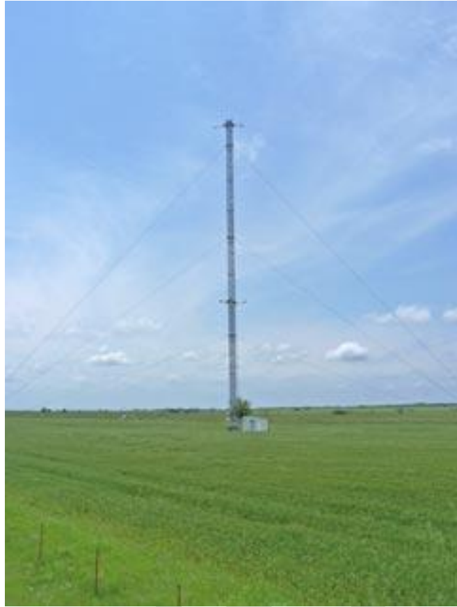
Figure: 4.B.1.A – Typical Temporary Meteorological Tower
