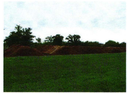
Figure 3. Compacted clay composting pad
