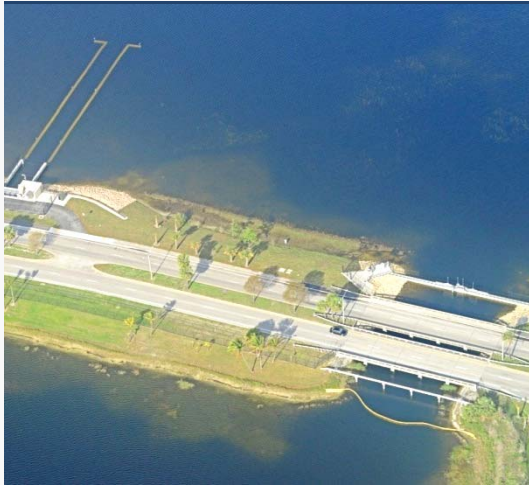
Clear Lake Divide Structure and Pump Station
