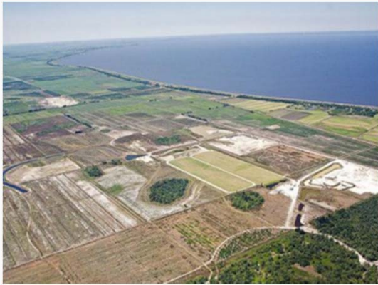
Above ground reservoirs to store surface water (Lake Point and C-51)
