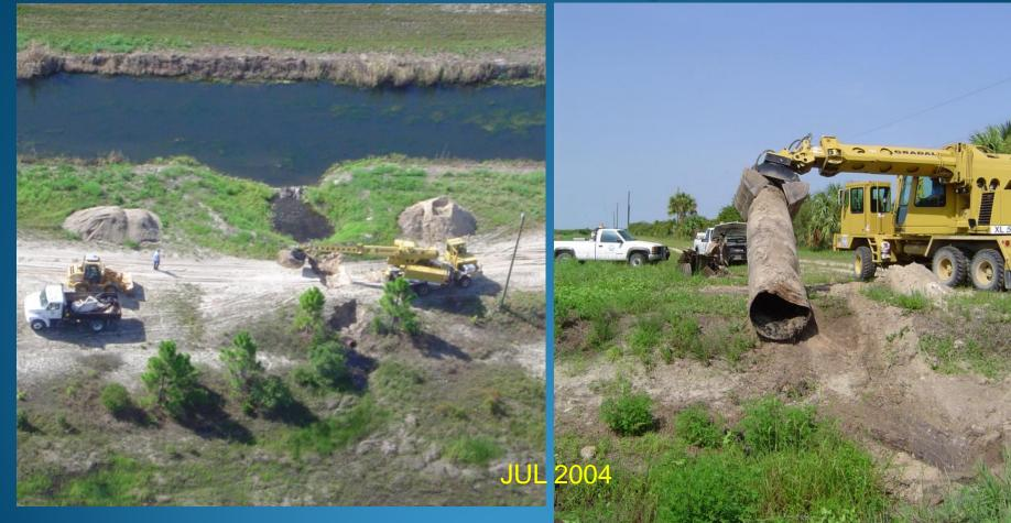
OCON TRACT – ALL 7 OLD CULVERTS REMOVED ALONG THE 1.75 MILE EASTERN EDGE: 4 WERE PLUGGED, AND 3 WERE REBUILT WITH NEW MATERIAL
